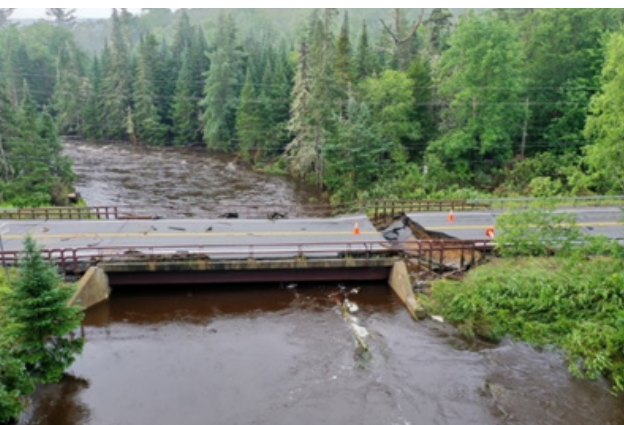
Flooding in July 2023 washed out this bridge over Fishing Brook between the towns of Newcomb and Long Lake. Photo courtesy of Discover Newcomb.
