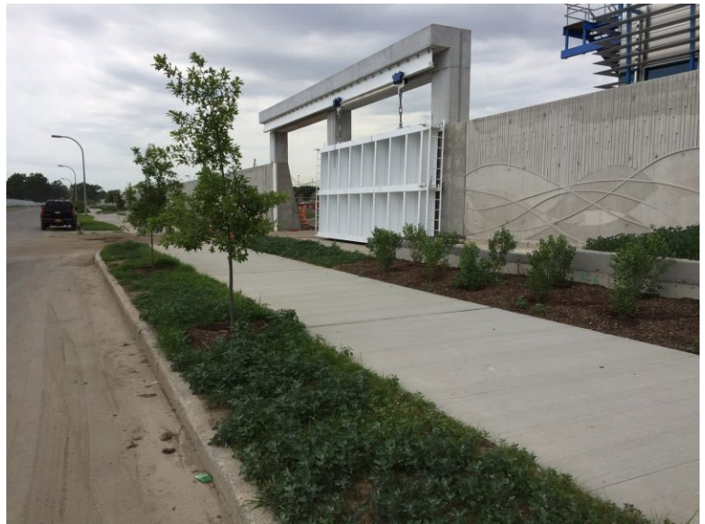
A perimeter flood protection berm and wall installed after Superstorm Sandy at the Bay Park Sewage Treatment Plant in Nassau County. Photo courtesy of Haugland Group.
